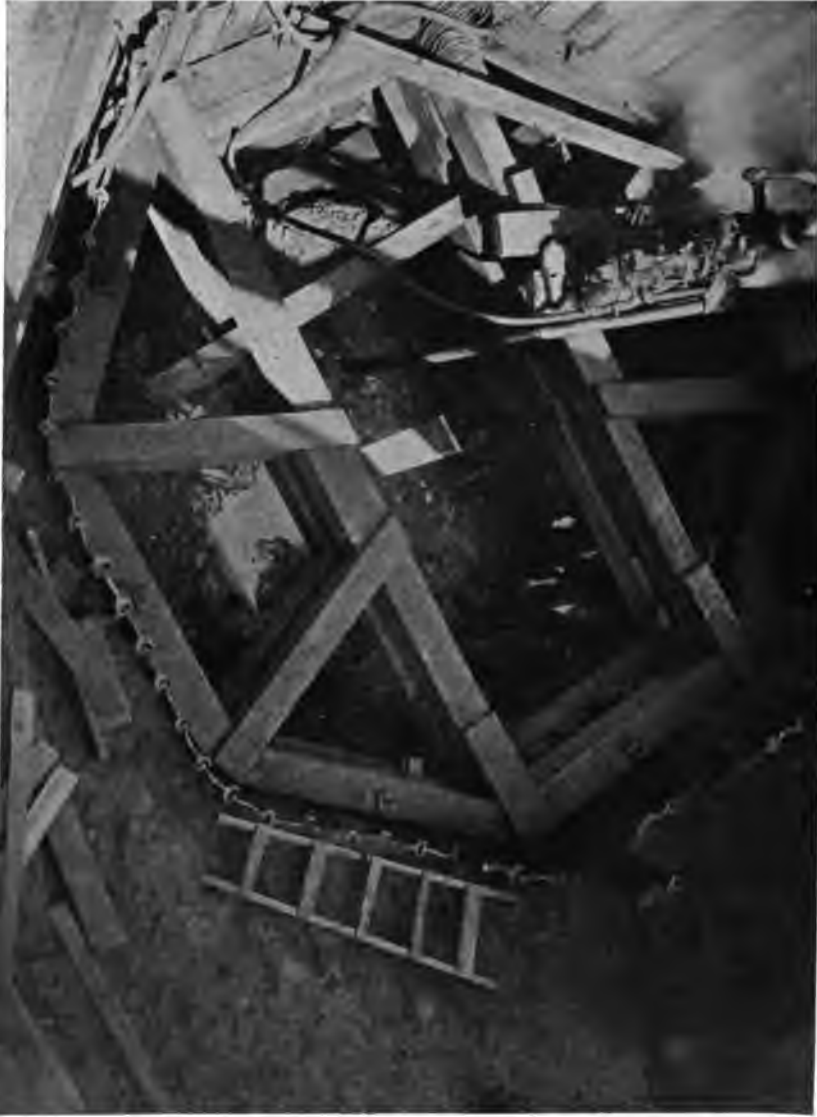
PLATE 207.—Shaft 5. City Tunnel. View Showing Framework and Steel Piling in Position.
